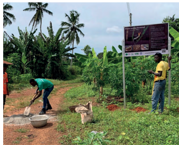
Signage being installed to raise awareness and direct visitors to White-necked Picathartes sites
